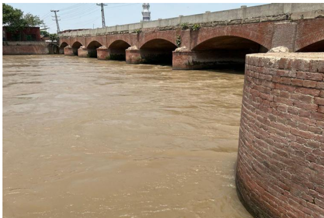
Figure 1. Picture of Khanpur canal
